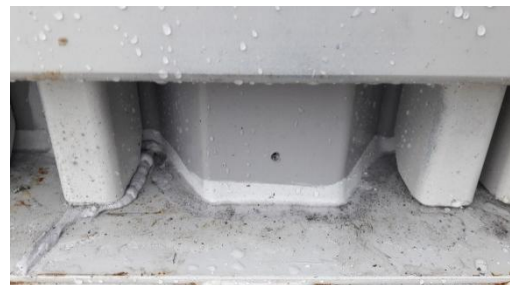
Photo 4.2 Sealant on edges sheet pile sections
