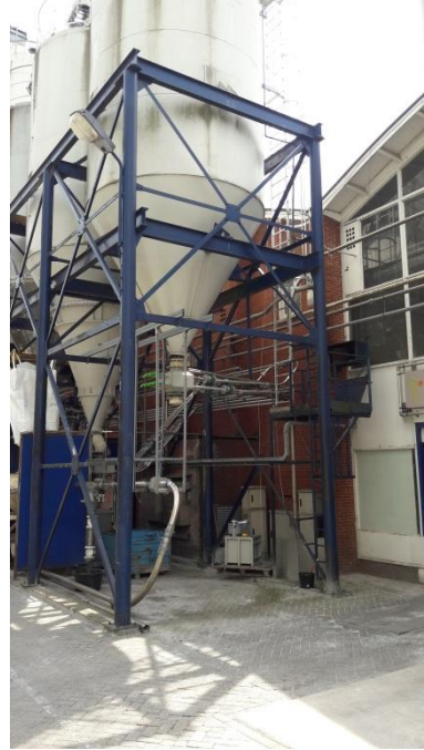
Photo 3.6 Height variation with ladder next to silo
